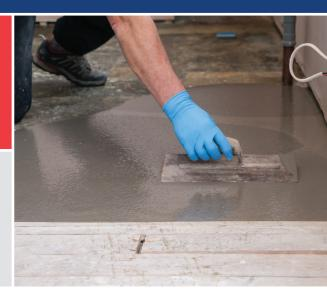
**SETCRETE™ DEEP BASE** is designed to raise floor levels quickly and economically and for smoothing uneven floors in light to heavy-duty internal applications. The versatility of the product allows for application between 5–50mm in one application.
