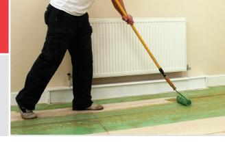
SETCRETE™ ACRYLIC PRIMER prevents unacceptably rapid drying of Coverage SETCRETE™ FLOOR LEVELLING COMPOUNDS over absorbent subfloors, and promotes adhesion to non-absorbent surfaces. It is suitable for use over normal underfloor heating installations and is coloured green to provide the user with visual control of coverage uniformity.
