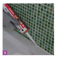
• All perimeters must be sealed using a waterproof silicone sealant.
