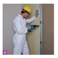
• Fix 12.5mm Glasroc H TILEBACKER or Gyproc moisture resistant grade plasterboard to all framing members at 300mm centres, using the appropriate length British Gypsum Drywall Screw, to give a minimum 10mm penetration into the stud.
