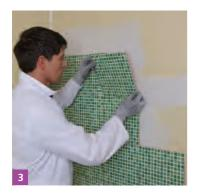
• Install tiles using a thin bed of adhesive, strictly following the manufacturers' recommendations. Ensure all screw heads are filled with adhesive.
