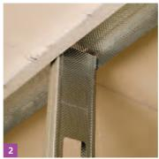
• Cut studs to a neat fit (maximum possible entry into head and base channel). The engagement should be a minimum of 20mm, allowing for any deflection where required.
