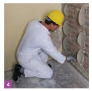
• Apply a continuous band of Gyproc Dri-Wall Adhesive at skirting level.
