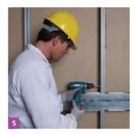
• When medium weight fixtures will be installed, for example a shower unit, install Gypframe 99 FC 50 Fixing Channel to accommodate the fixture.
