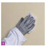
• Ensure the boards are dust free prior to installation of the tiling system.
