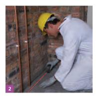
• Mark chalk lines to the floor and ceiling to indicate the positioning of the Gypframe GL8 Track.
