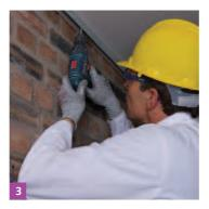
• Fix Gypframe GL8 Track to perimeters, with the longer leg towards the lining, at 600mm centres using the appropriate fixing.
