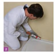
• The perimeter of the wall, e.g. base, head and wall abutments, should be sealed with a silicone-based sealant.
