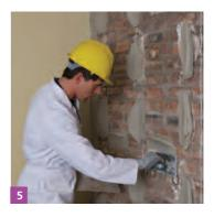
• Apply horizontal dabs of Gyproc Dri-Wall Adhesive at mid board height to support tile loading.
