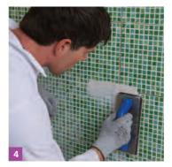
• Once set, ensure tiles are fully sealed using a waterproof grout.
