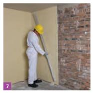
• Tap the board back firmly using a straight-edge until it aligns with the ceiling and floor chalk lines.
