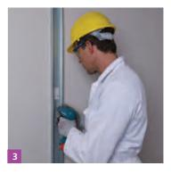
Locate the first stud, twist into position and fix to the abutting wall at 600mm centres
