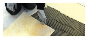
You can tile directly onto the pre-primed surface, but wipe down to remove any dust before you start.  Seal around any perimeters (including the board base) with waterproof silicone sealant. Fill joints with waterproof tile adhesive.
