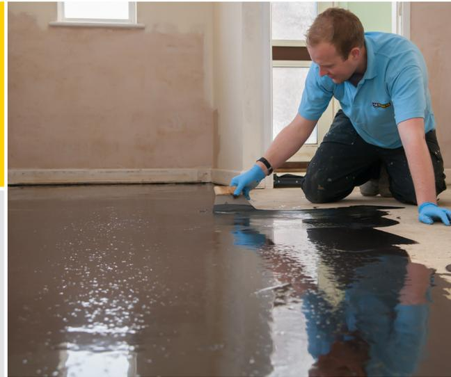
**SETCRETE™ RAPID SET DPM** is a solvent free, two part epoxy resin system which cures to provide a damp proof membrane. SETCRETE™ RAPID SET DPM provides a barrier to residual construction moisture and rising damp, preventing moisture from adversely affecting subsequent floorcovering installations. The product is applied in one coat and has a curing time from just 3 hours, allowing early installation of floorcoverings in fast track building programmes.
