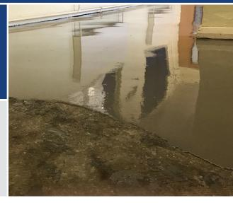
**SETCRETE LEVEL-SMART** is designed for preparing sound internal subfloors prior to the installation of new floorcoverings and can be applied at thicknesses from 2-30mm. It is particularly suitable for direct application over old adhesive residues (such as bitumen and carpet tile tackifiers) without the need for priming. Its fast setting characteristics enable a walk-on time of just 90 minutes and new floorcoverings can be installed from 4 hours.
