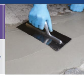
**SETCRETE<sup>TM</sup> CONCRETE REPAIR** is an easy to use, single component, Polymer Cement Concrete (PCC) mortar for the non-structural repair of damaged or worn concrete. It is suitable for use on both internal and external applications and can be applied to horizontal and vertical concrete surfaces.
